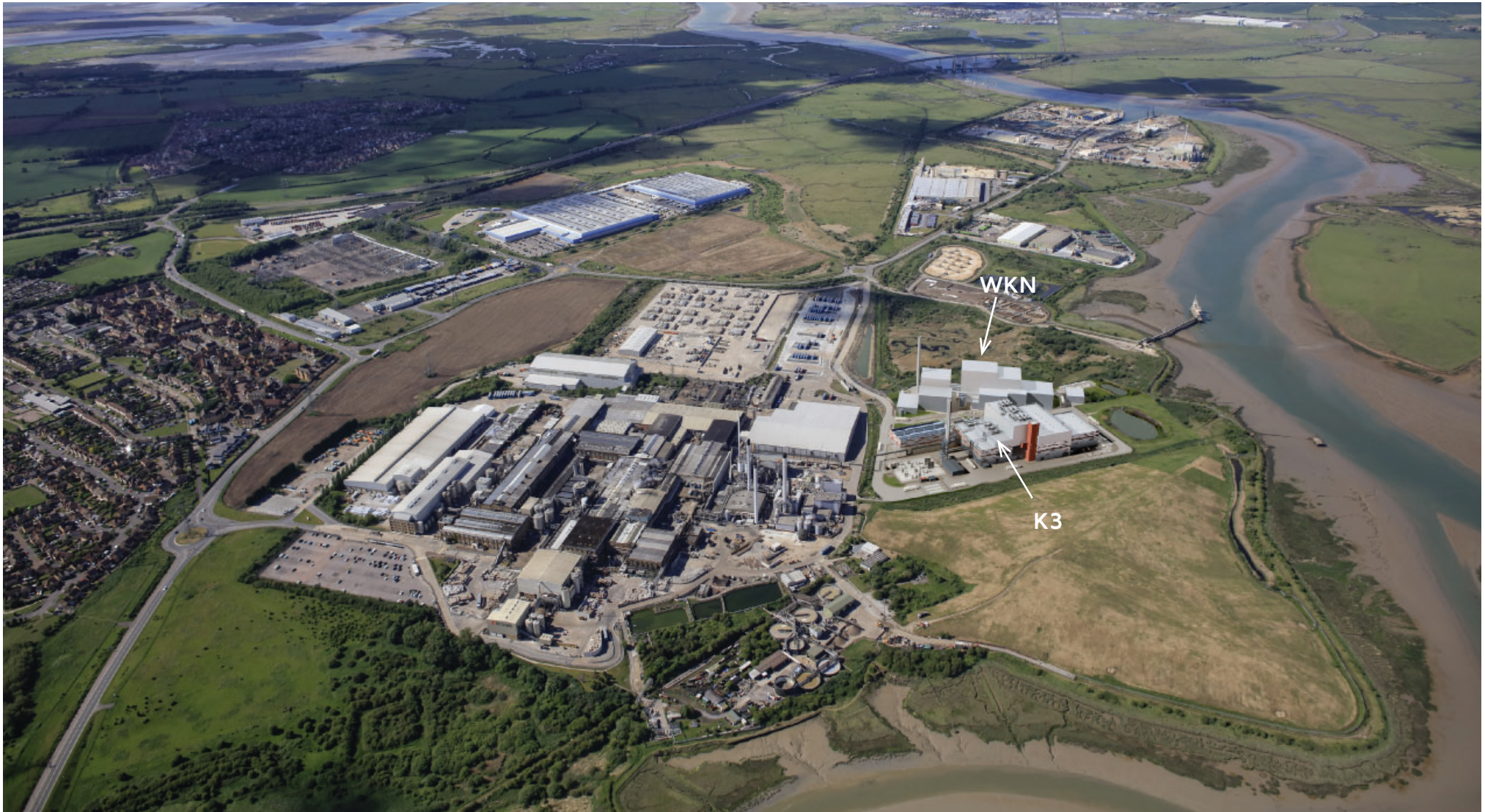
Figure 20.1: Aerial view showing the K3 and WKN developments in context
